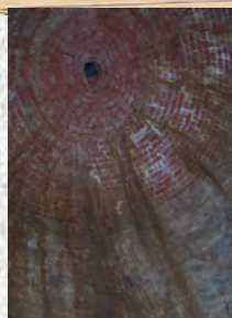
This is view of the cistern looking up from inside the cistern.
