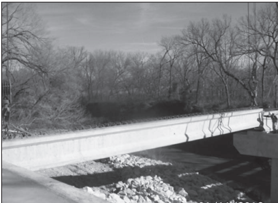
Concrete beams form the foundation of the bridge. Picture taken Jan. 11, 2012.
