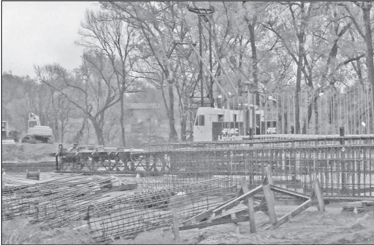
Materials used to create the new bridge.
