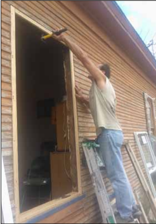
Ronnie Cooper removes and reframes old inefficient windows.
