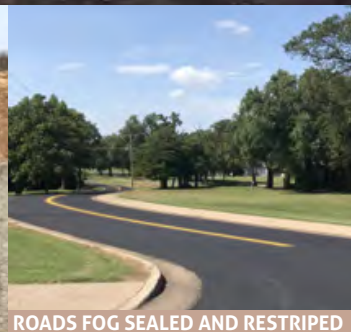
ROADS FOG SEALED AND RESTRIPE
