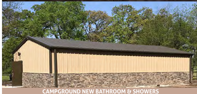
CAMPGROUND NEW BATHROOM & SHOWERS
